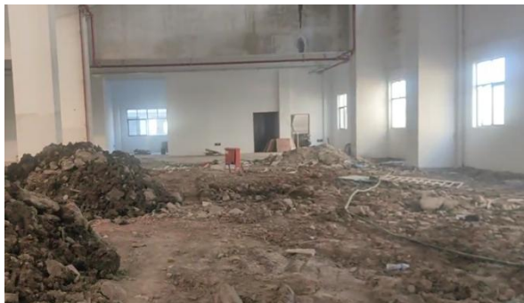
探伤铅房拟建址北侧
